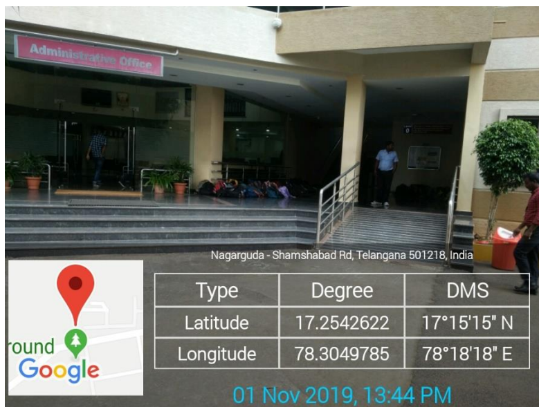
Block-1 Ramp and Hand Rails
