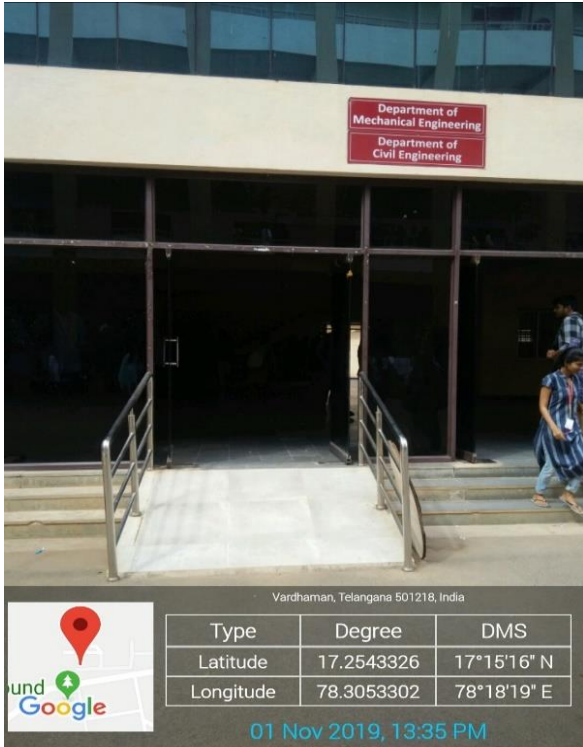
Block-2 Ramp and Hand Rails
